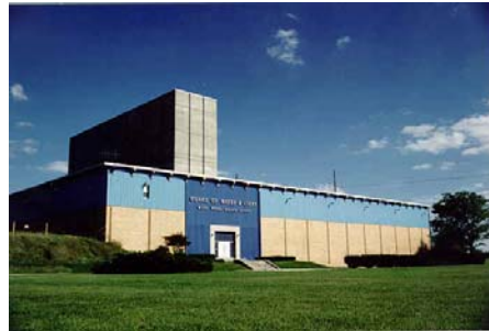
Water Conditioning/ Treatment Plant
