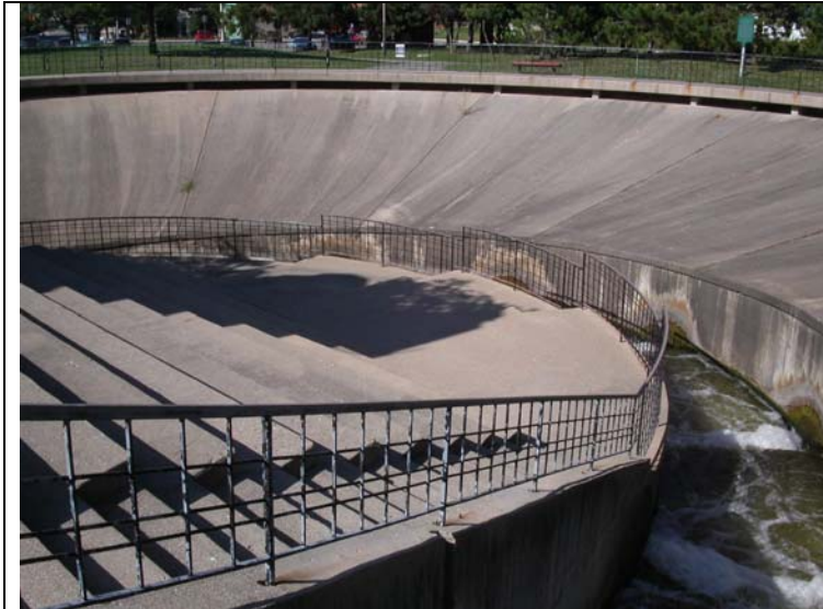
Brenke Fish Ladder
